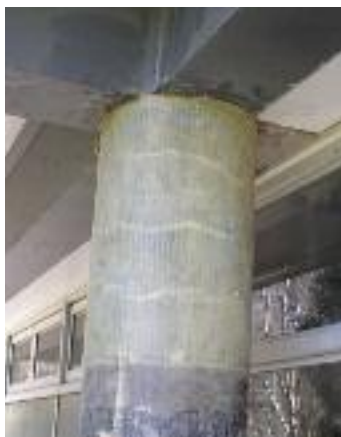
Just five days before the September earthquake, BBR completed the strengthening of 23 circular columns at the University of Canterbury's Student Services Building.
