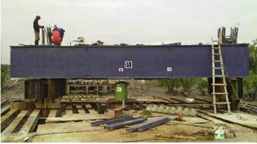
SUNGAI SIOL BRIDGE, MATANG, SARAWAK, MALAYSIA
