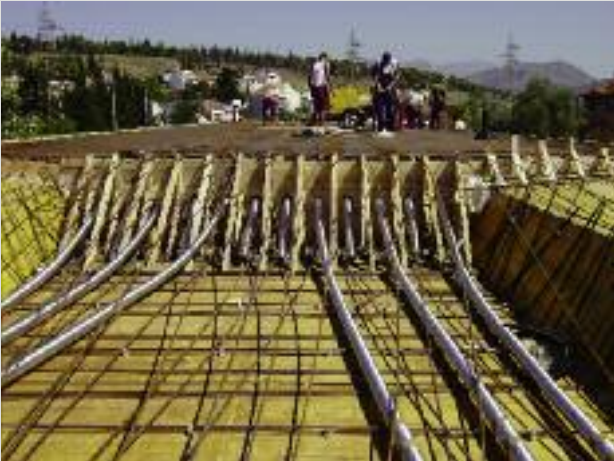
RIBNICA BRIDGE, PODGORICA, MONTENEGRO
