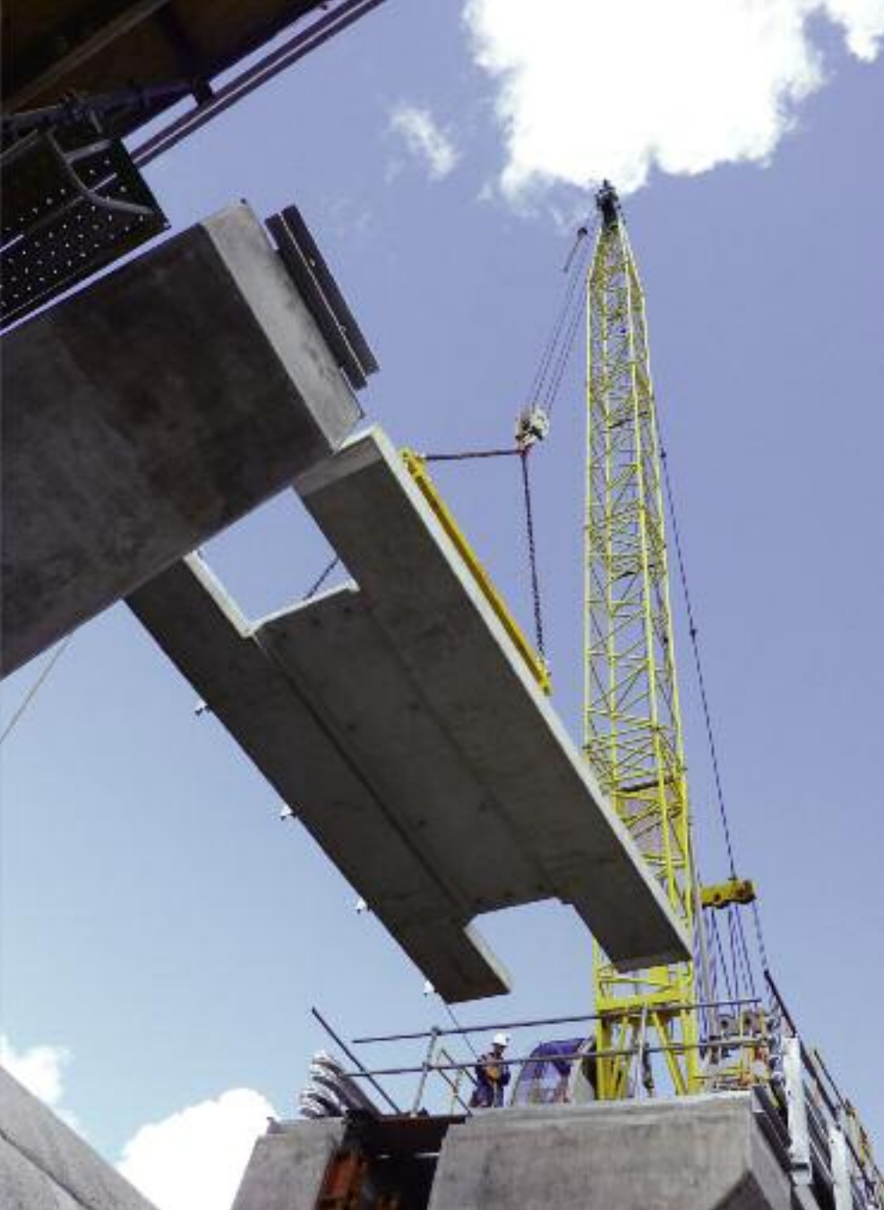
WELLINGTON DAM, COLLIE, WESTERN AUSTRALIA
