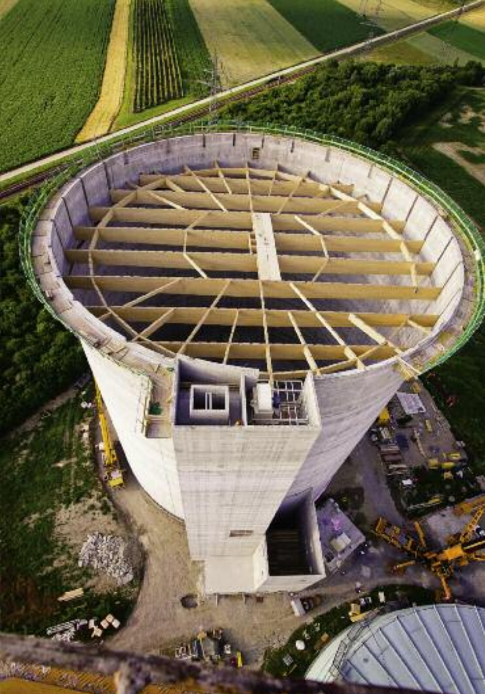
SUGAR SILO, TULLN, AUSTRIA
