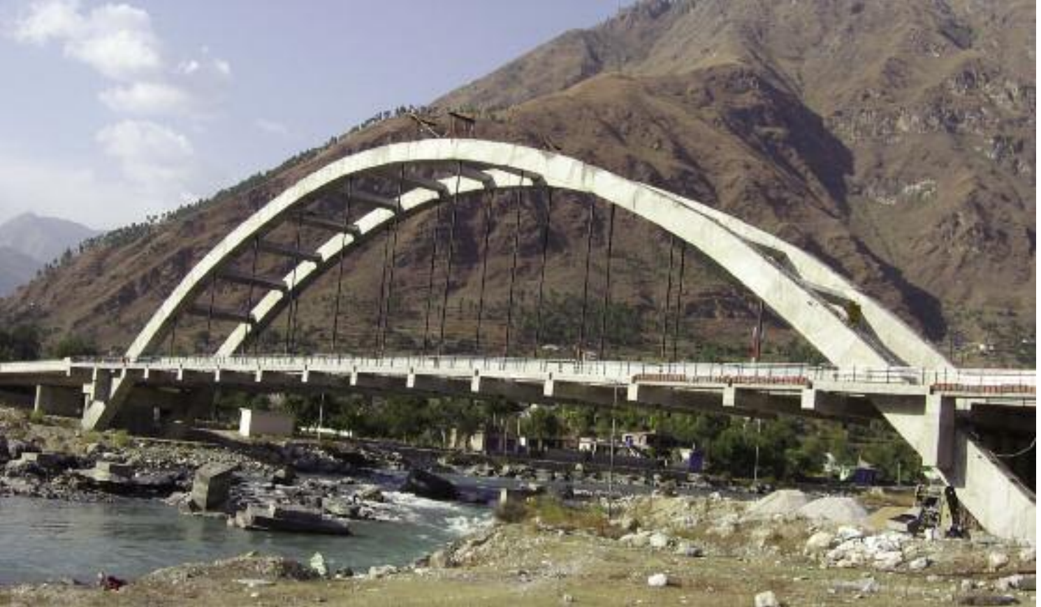
PARVATI RIVER BRIDGE, HIMACHAL PRADESH, INDIA
