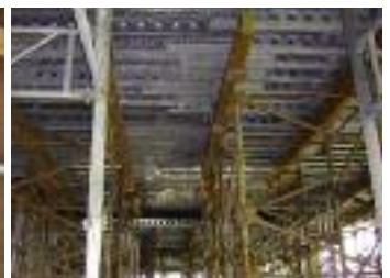
Heavy duty scaffolds to support half of total concrete weight
