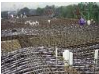
All beam tendons installed before first stage casting
