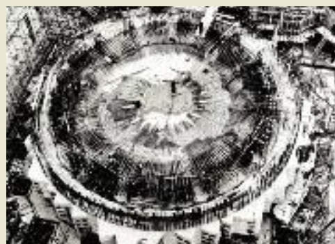
ABOVE: Construction of bottom cap with buttresses for anchorages of the UK's Dungeness B pressure vessel. BELOW: Testing of BBR anchor head. Stressing device consists of three 500t jacks, hydraulic pumps and load cells.
