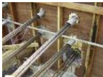
Stage 1 tendons stressed and forces in props released before Stage 2 casting
