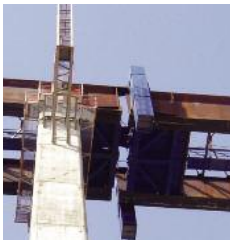
BBR S-750 pulling jacks were used during the last phase of launching.
