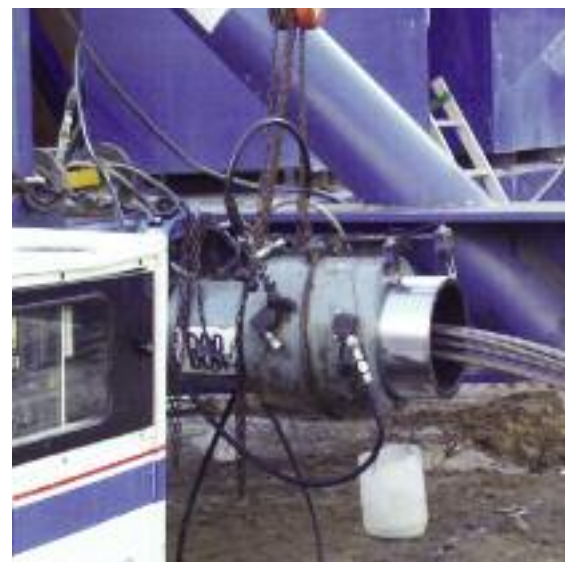
BBR S-750 pulling jacks were used during the last phase of launching.
