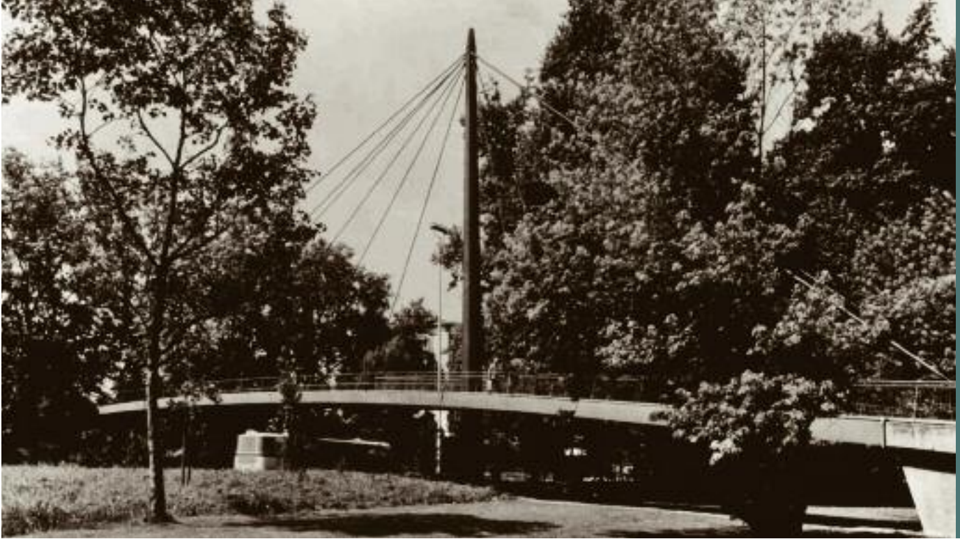
In 1961, the first bridge to be built using parallel wire cables was the pedestrian Schillersteg Bridge across the Schillerstrasse in Stuttgart, Germany.
