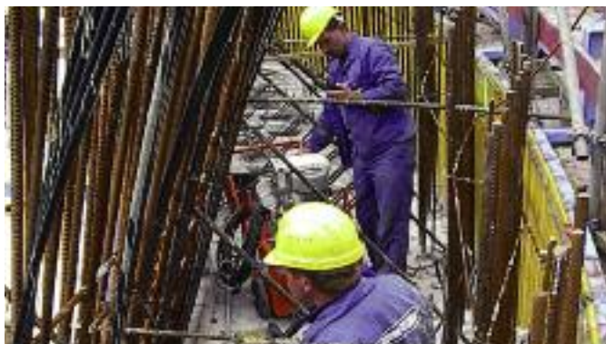
Tensioning of the conic prestressing tendons with VT 1000 prestressing jacks.
